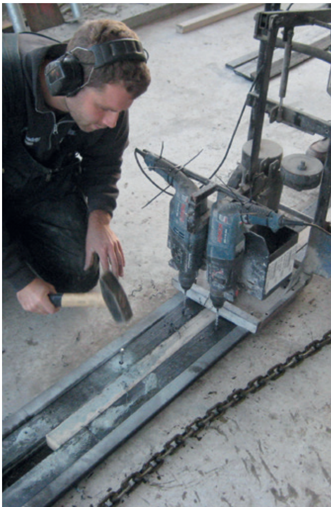
Figure 2: Mounting of the plastic rail
