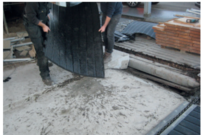
Figure 3: Laying the rubber mats
