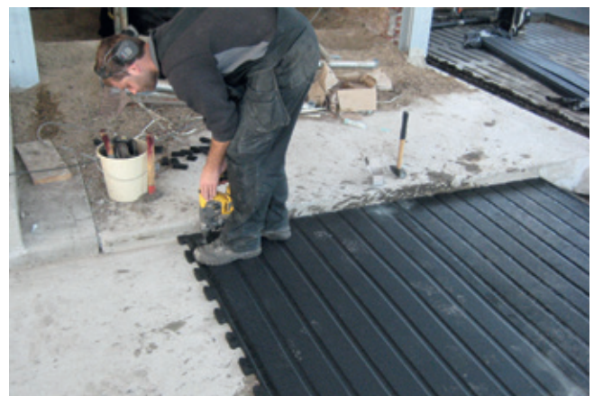
Figure 4: Attachment of the rubber mats
